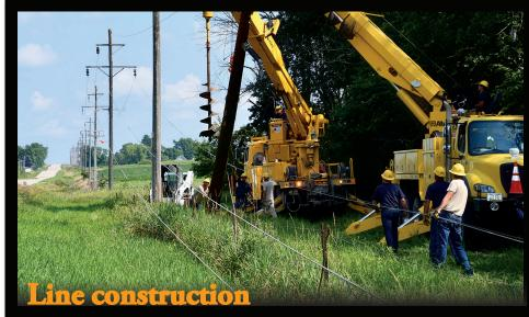
**Above** Corn Belt Power transmission crews work south of Highway 3 on the Parkersburg-to-Bristow line rebuild. Crews will replace 147 poles along the 10-mile stretch, while also replacing old wire with more robust conductor.
